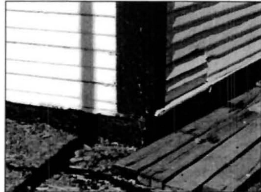
Avoid wood-soil contact, as moisture will damage heritage building fabric.
