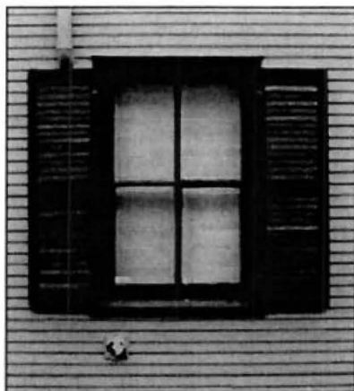
Original window openings and features, such as the windows, trim, sillas and shutters shown here should be protected and maintained.
