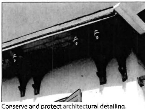
Conserve and protect architectural detailing.
