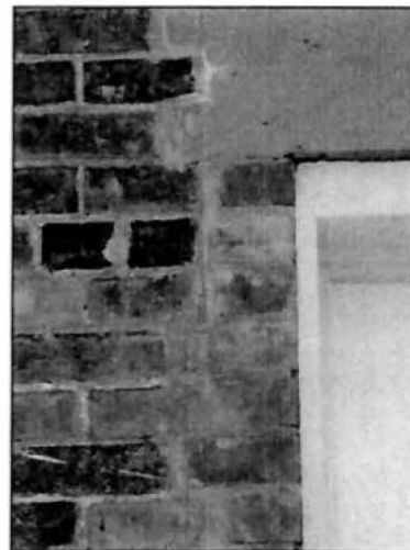
Repointing should avoid the use of Portland cement (as shown above) in favour of a lime-based mortar mix.
